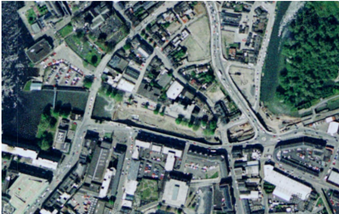
Plate 14-12. OSI aerial photography from 2000 showing works in the Abbey River associated with the Limerick Main Drainage Project.
