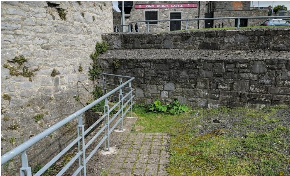
Plate 14-57. King John's Castle, National Monument, RPS 004, showing existing railings, to be replaced with glass panels, with tie into the later wall to the right
