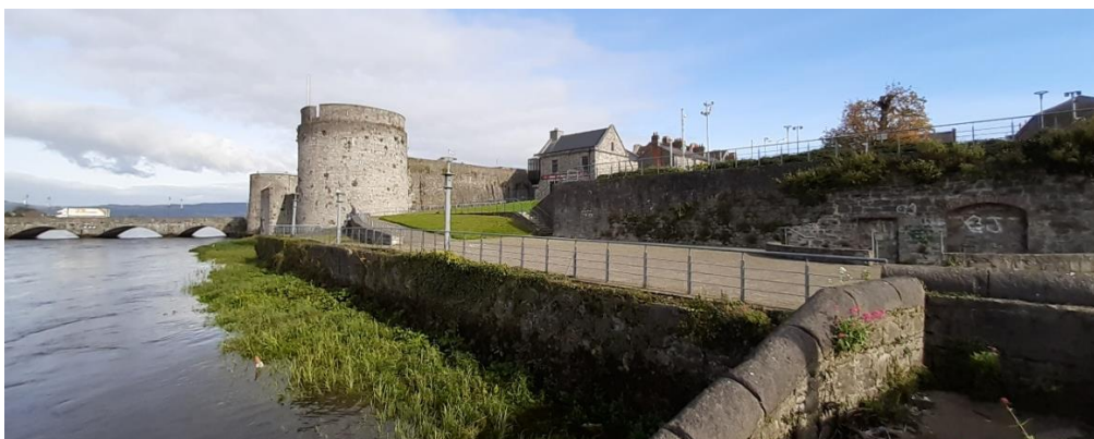
Plate 14-45. View to the north to King John's Castle, with steps to foreground, undercroft cellars to the right
