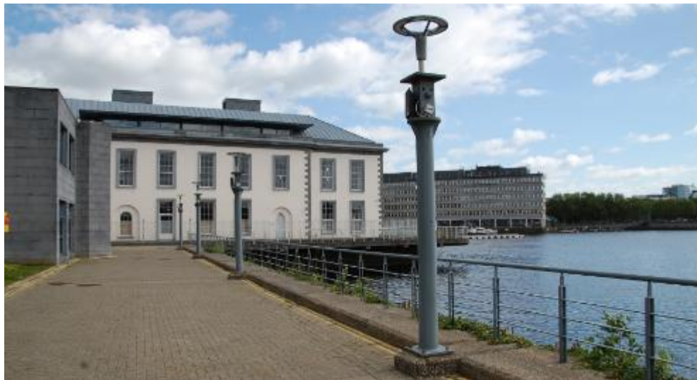
Plate 14-47. County Court House, from north, showing board walk and railings, along northern and western sides
