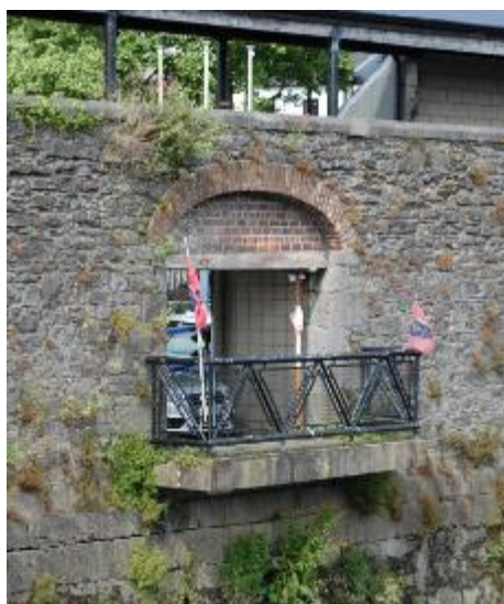
Plate 14-59. Opening in south wall
